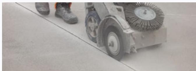
Joint brush used in road construction
